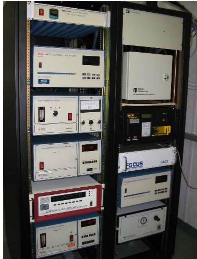
Above - Air Quality Monitoring Instrumentation inside the Henry Pirker Air Monitoring Station
