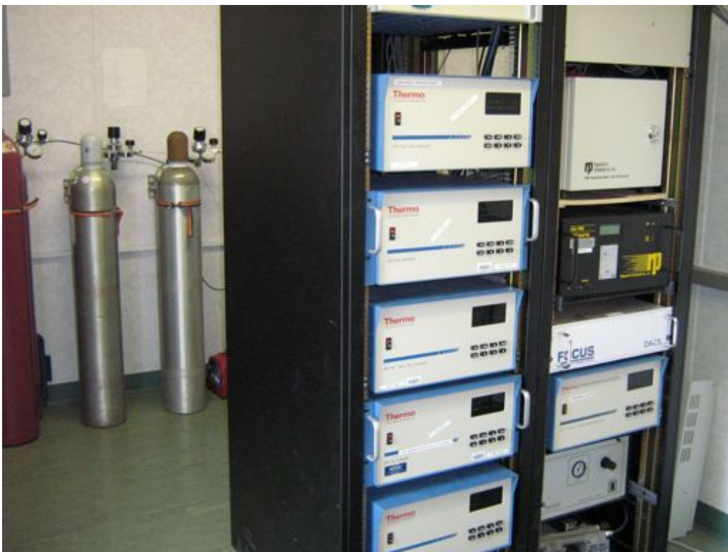
Continuous Monitoring Equipment inside Henry Pirker Station (Grande Prairie).
