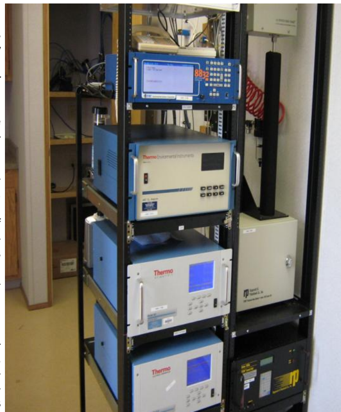
Inside the Beaverlodge Air Quality Monitoring Station
