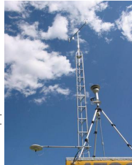
Continuous Monitoring Station Meteorological Equipment
