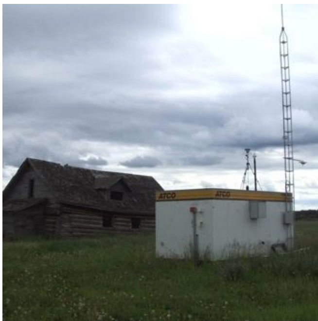
Smoky Heights Station was relocated during monitoring period.
